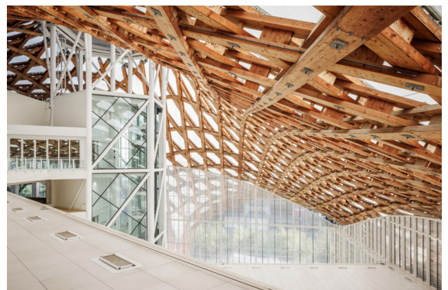
Centre Pompidou - Metz
